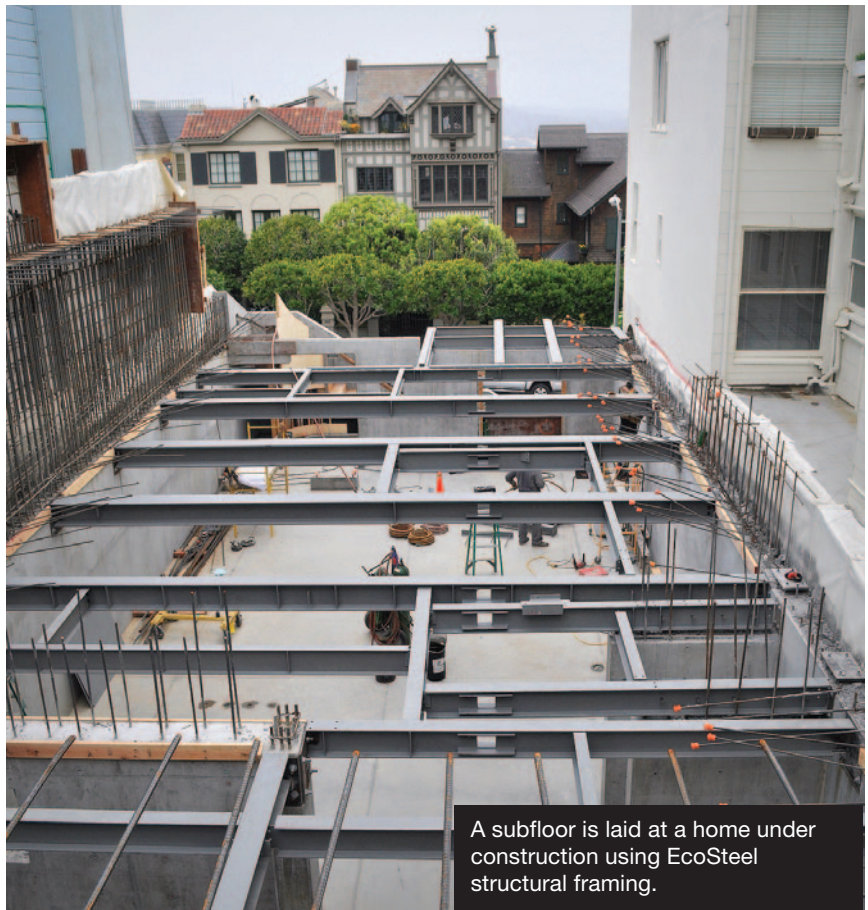
EcoSteel produces a prefabricated kit of parts that is assembled on the building site.
