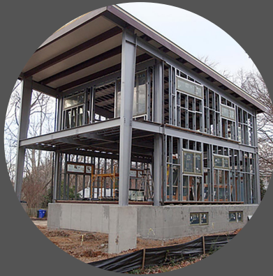
BOLTED STEEL STRUCTURE
